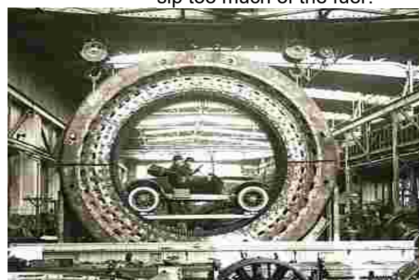
PR pic from 1919 when ASEA built a world record generator. A car fitted inside its stator.
